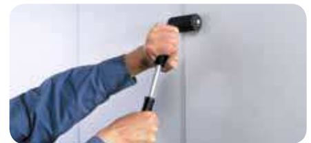
Remove the liner, fit the two surfaces together carefully and apply more pressure to form a bond.
