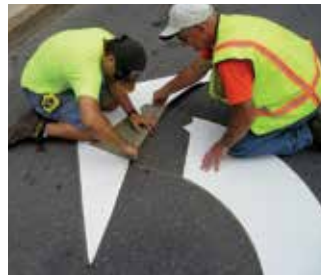
Clean, lay out and adhere
