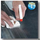
Simply clean with a solution of 50:50 water and isopropyl alcohol and wipe dry. Using 3M Adhesion Promoter AP111 is recommended after cleaning for maximum performance.
