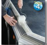
Roll down with a soft roller to conform over contours, seam edges, rivets or screw heads.
