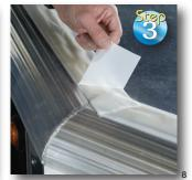
Peel off the release liner.
